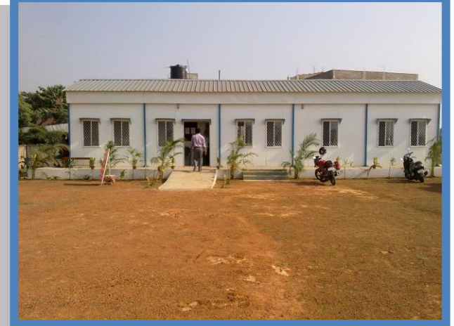
Burdwan Health City Project at Goda. The project cost of the 1 st phase of the project is 250 crores
